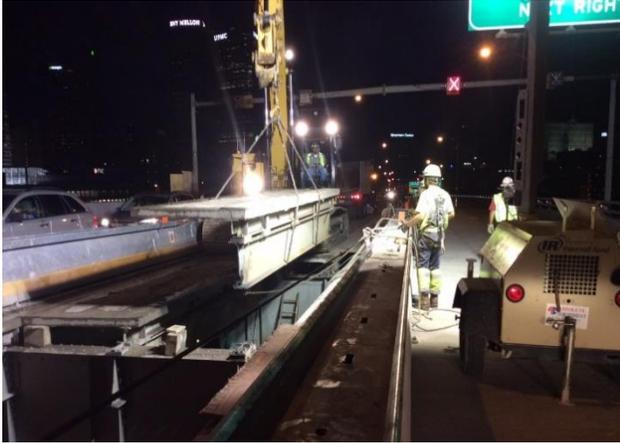
**Figure 7:** Removal of existing stringer with section of deck during nighttime lane closure
