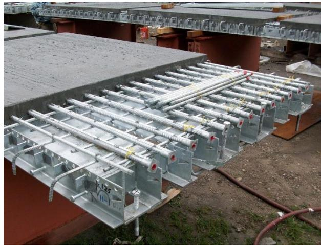
**Figure 4:** Exodermic grid deck panel with reinforcement bars and precast panel zones
