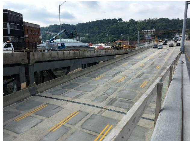
**Figure 8:** Completed precast Exodermic grid deck section showing CIP concrete joints (lighter)
