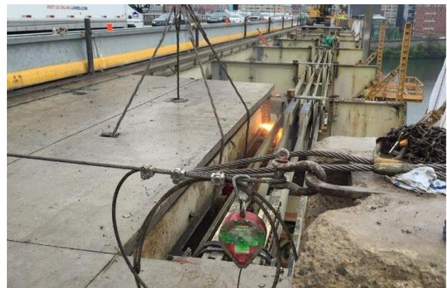
**Figure 6:** Preparation of the existing deck for removal: torch cutting stringer ends
