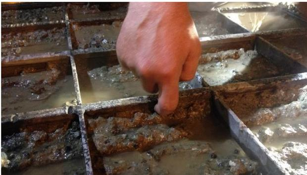
**Figure 3:** existing grid deck condition following hydro-demolition
