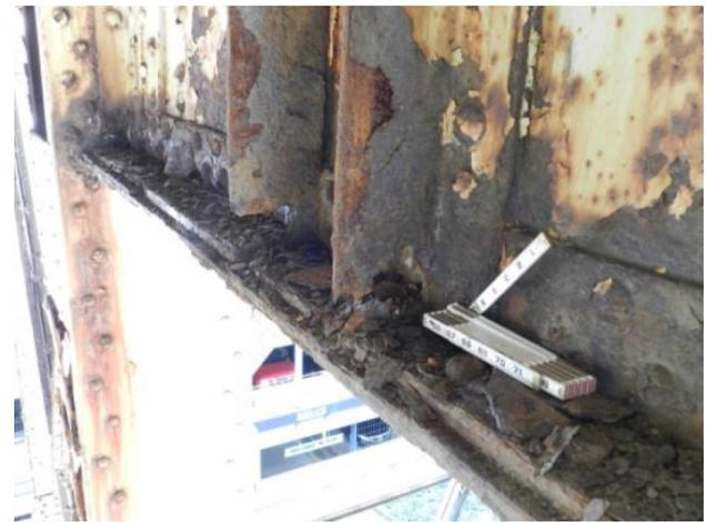
**Figure 2:** typical superstructure condition at leaking joint.
