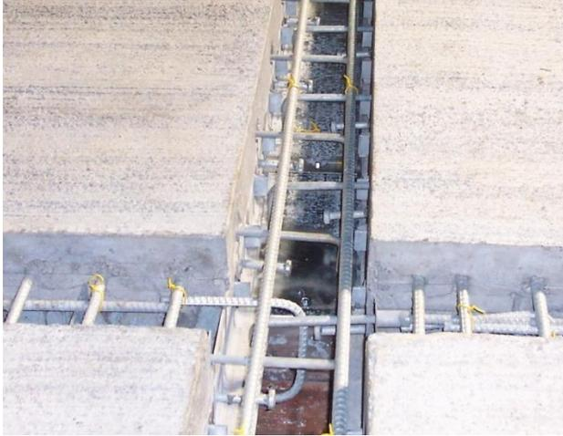
**Figure 5:** Exodermic grid deck panel with precast zones assembled on the bridge
