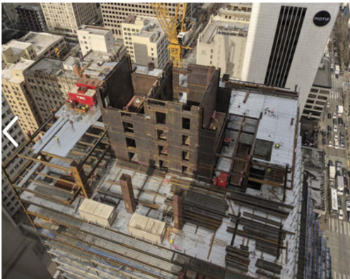
(a) Speedcore erection for Ranier Square (Seattle, MKA)
