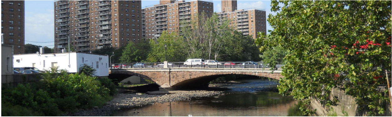
Figure 2 - First USA Melan bridge – West Broadway over Passiac River, Paterson City, NJ.
