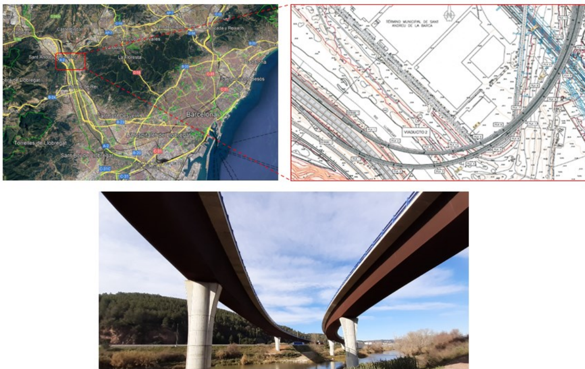
Figure 1. Location and general view of PR-04-B015 bridge
