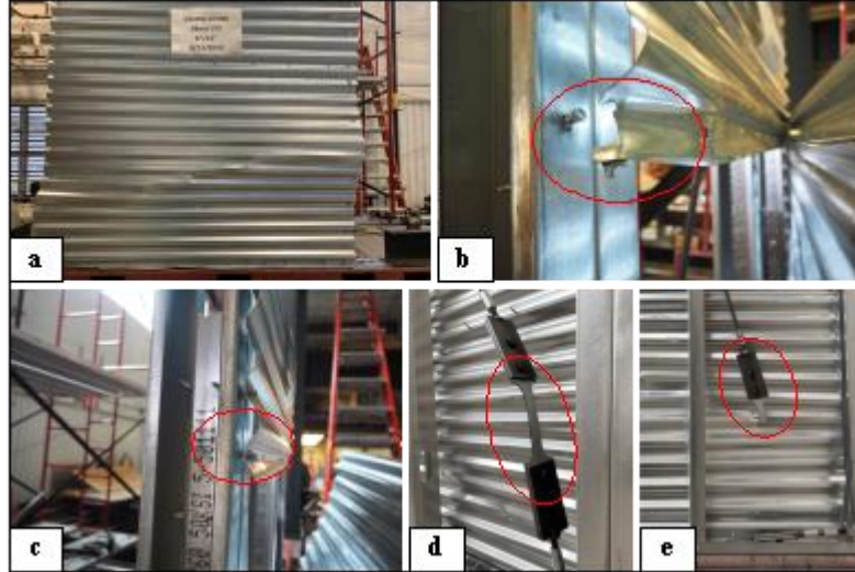
Figure 11 Failure modes of shear walls with EDB (a) sheet buckling (b) screw pulling over (c) screw pulling out (d) EDB yielding (e) EDB fracturing
