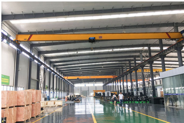
(c) Warehouse building with modular steel frames containing stepped crane columns (from finework-cranes.com)
