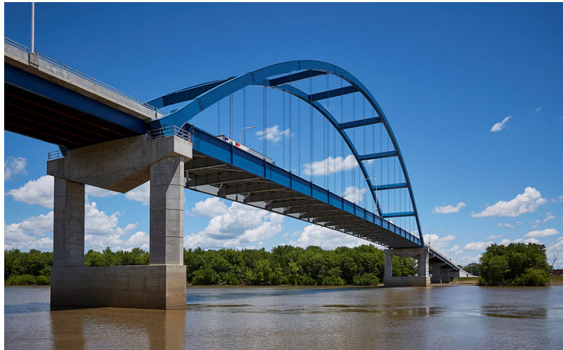
Fig. 5: Tied arch bridge designed using the Direct Analysis Method (courtesy of Shankar Nair, EXP Design)
