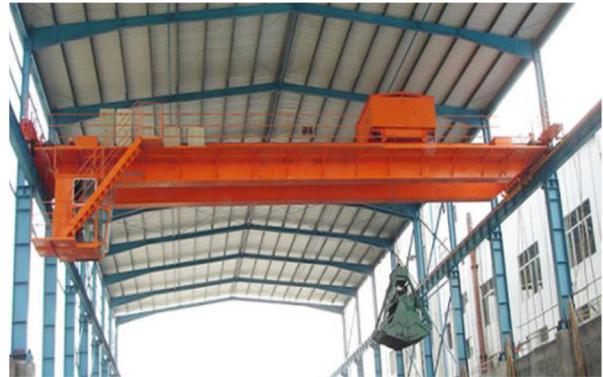
(b) Crane support structure with gabled portal frames and stepped crane columns (from ellsenbridge-crane.com)
