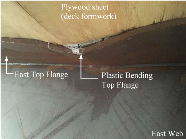
Figure 16 – Offset Top Flanges Plastic Bending – Tub 2
