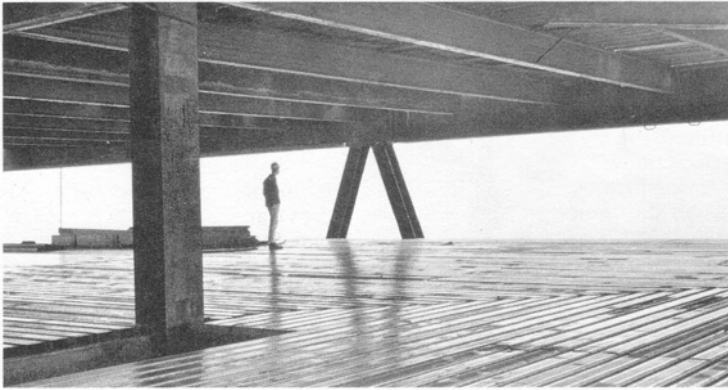
Floors are column-free between core columns (left) and the exterior. Note the absence of intermediate exterior columns at this level, which is immediately below the apex of a wind bracing triangle. Here the floor beams (top) frame into plate girders.
